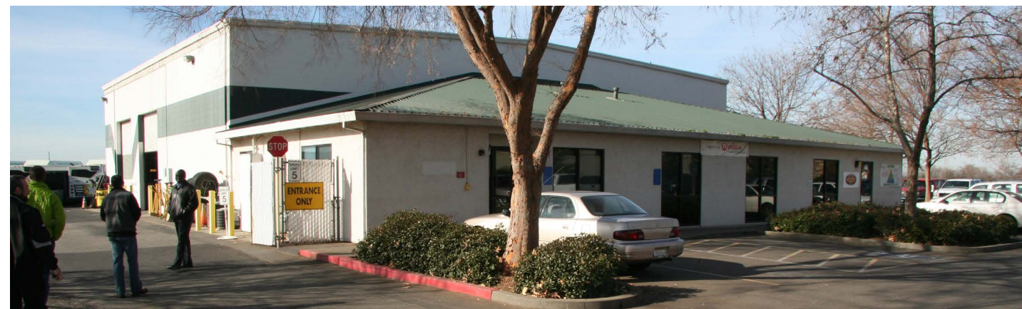
Existing B-Line administrative and maintenance facility.
